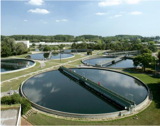
Municipal and industrial water treatment
