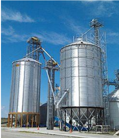
Grain/rice/Wheat/Seed hopper – Controlled atmosphere storage using carbon dioxide
