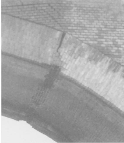
Fig. 1 - Plastic hinge developed in the arch barrel of a collapsed bridge on the Scrivia river (Alessandria, Italy).
