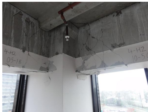
Figure 6: Beam plastic hinges in a 22-storey reinforced concrete building constructed in mid-end 1980s (currently under demolition). Top Left; photo of building under construction (courtesy of Restrepo).
