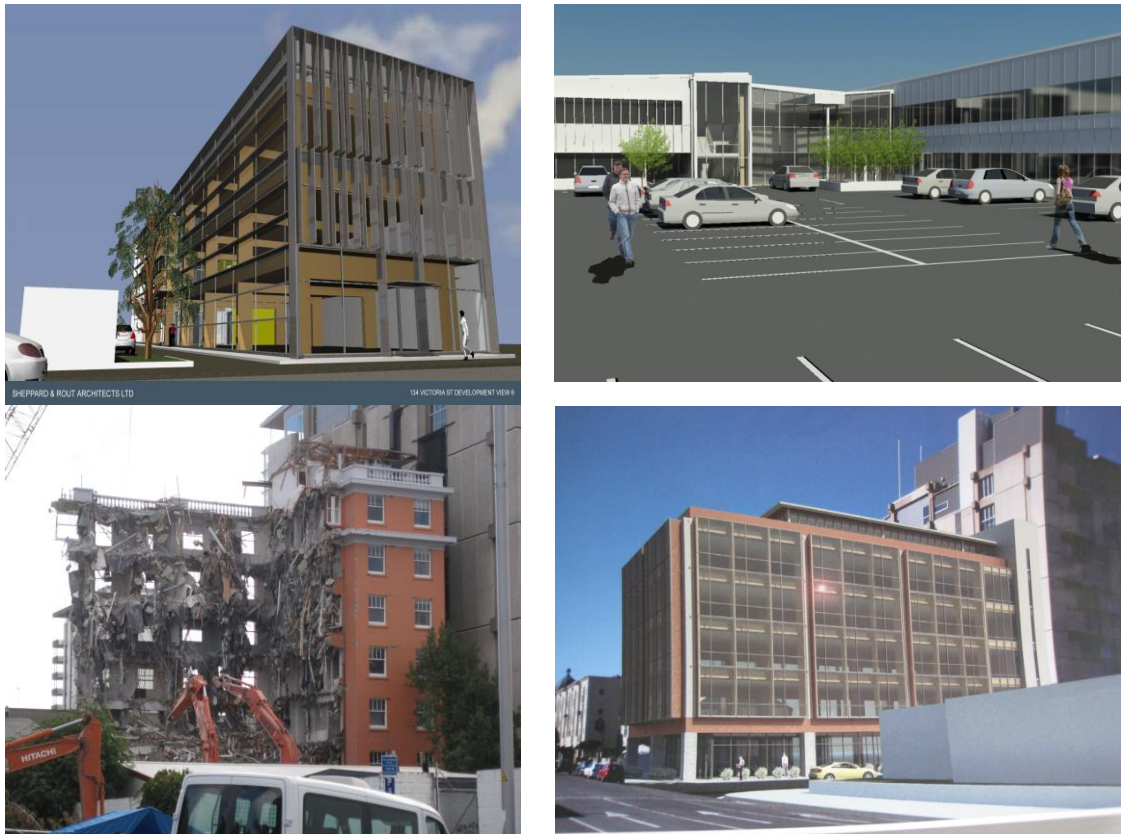
Figure 36: Christchurch Rebuild: several Pres-Lam buildings in the final stage of their design or under current construction. Top left: Merritt Building, Structural Engineers: Kirk and Roberts; Architects: Sheppard and Rout; Top Right: Trimble, Architecture and Structures from Opus International (Brown et al., 2012); Bottom Left: St Elmo Courts a 1930 RC building demolished; Bottom-right: rendering of the “new St. Elmo” using a combination of base-isolation and a post-tensioned timber-concrete two-way frame in the superstructures, Architect: Ricky Proko, Structural Engineers: Ruamoko Solutions.
