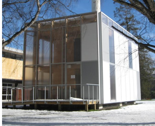
Figure 34: From laboratory specimen to office building: 3D Test Specimen tested in the lab (Newcombe et al, 2010), dismantled and reconstructed (Smith et al., 2011) on UC campus as EXPAN/STIC office.
