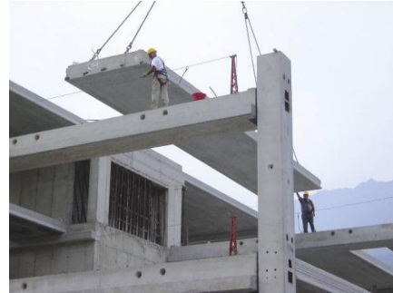
Figure 28: Application in Italy of the Brooklyn System, B.S. Italia, with draped tendons (Pampanin et al. , 2004).
