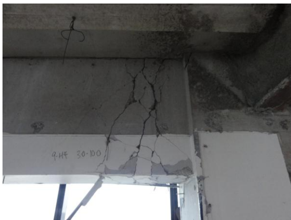
Figure 6: Beam plastic hinges in a 22-storey reinforced concrete building constructed in mid-end 1980s (currently under demolition). Top Left; photo of building under construction (courtesy of Restrepo).
