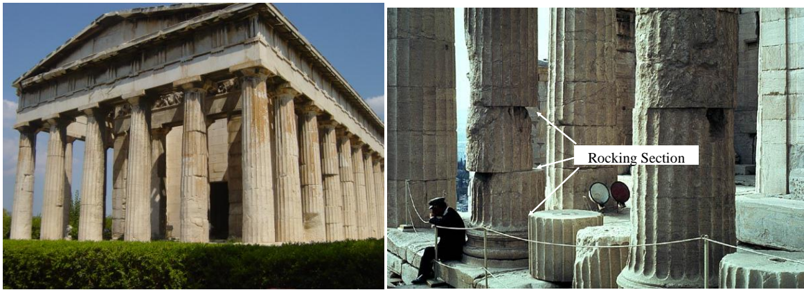
Figure 15: Examples of earlier implementation of rocking systems, self-centring and limited damage response under earthquake loading. Left: Dionysus temple in Athens, ancient agora, Right: Rocking segments of marble columns (Acropolis, Athens).
