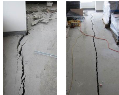
Figure 21. Beam elongation effects (after fib, 2003) and example of extensive cracking in the diaphragm topping of precast concrete floors within a multi-storey buildings following the 22 February 2011 Canterbury Earthquake.
