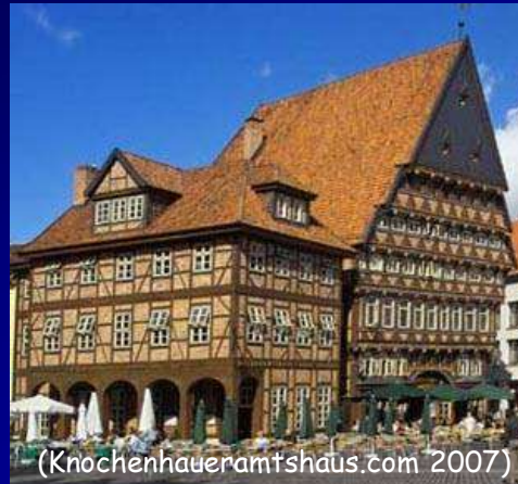
12th century Knochenhaueramtshaus, Germany 8 storeys standing 25.7m tall
