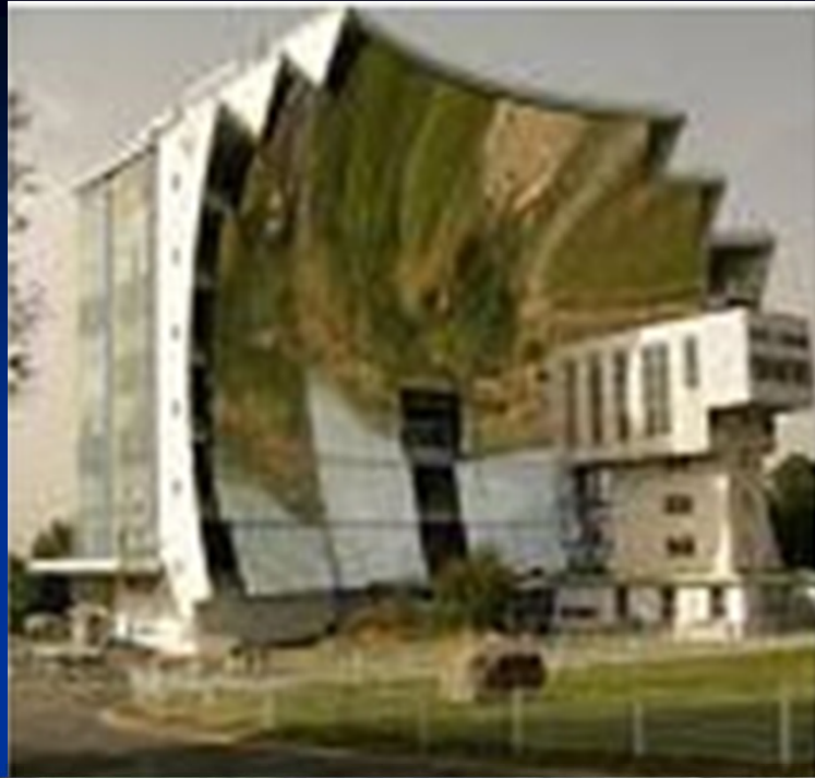
Four Solaire, Odeillo
