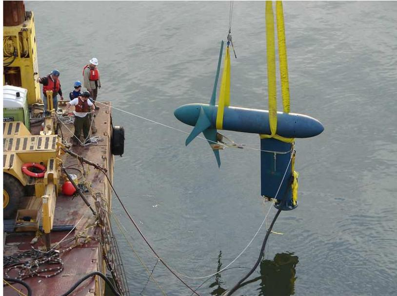
*Fig. 2.22 - Verdant Power Free-flow Turbine Being Deployed in East River (December 2006).*
