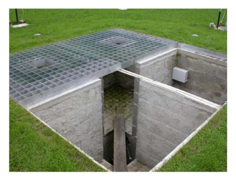
Fig. 4: The gratings, the pit internal walls and the pit recess for drainage (Vigna di Valle, Italy, 2007).
