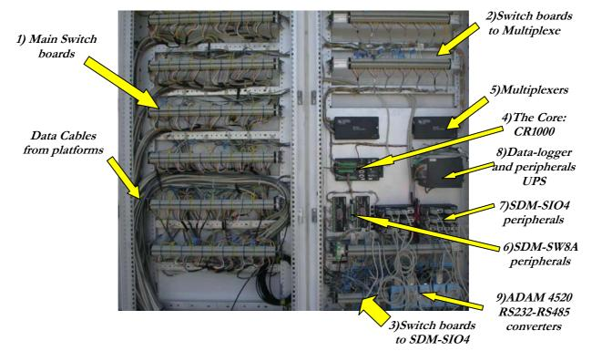
Fig. A - WMO Field Intercomparison of RI – Data Acquisition System
